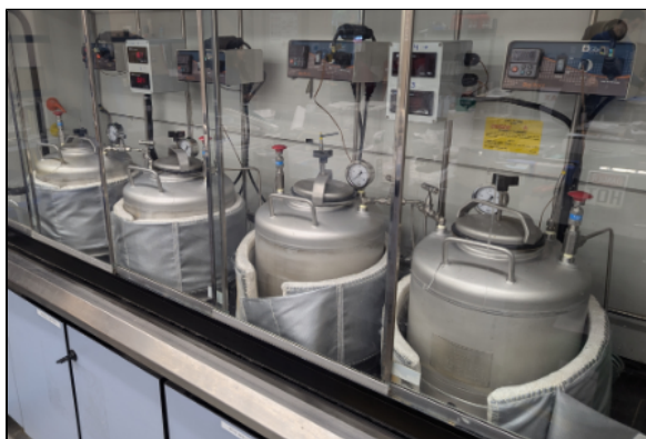
Sealed Heated Immersion Vessels
